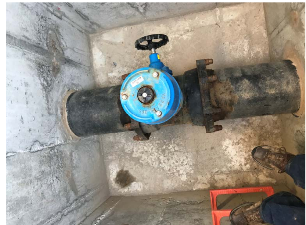
Interior arqueta F6-1U
