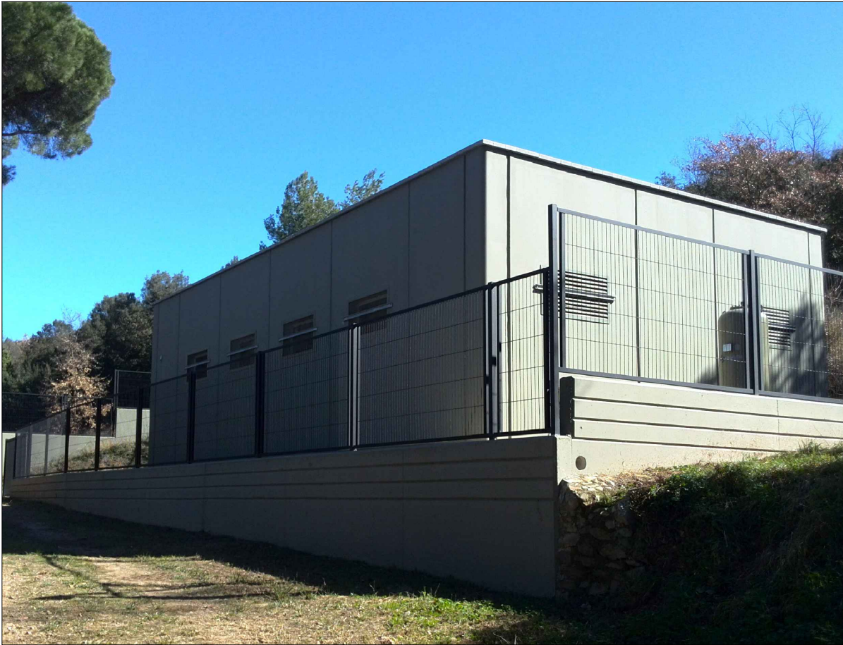
BOMBAMENT MONTORNÈS-CAN BOSQUERONS BV-5001, 6 08107 Martorelles UTM: 46849, 4598763
